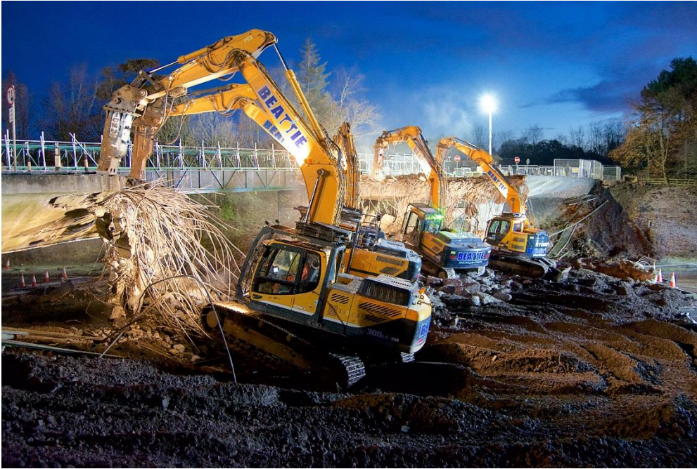
Beattie Demolition excavators demolishing the cantilever spans
