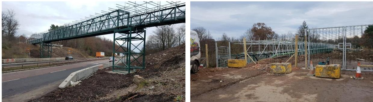
Prior to the demolition of the bridge, a temporary steel service bridge was constructed. This bridge carries Vodafone, Virgin Media and Scottish Power cables. The Council is currently exploring the possibility of opening this temporary bridge to pedestrians, however for the time being it is only suitable for access by maintenance personnel.
